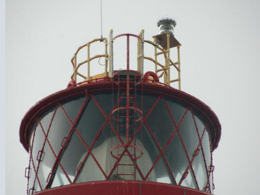
Right: New lantern roof arrangement with the 18 NM standby lantern and radar beacon (racon).
