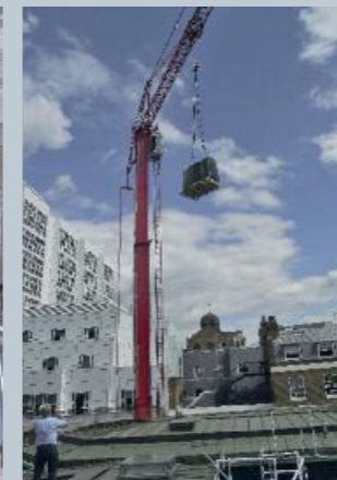
Above right: The unit is located in the roof top plant room which can only be accessed by removal of a section of the roof and via a small aperture in the structure.
