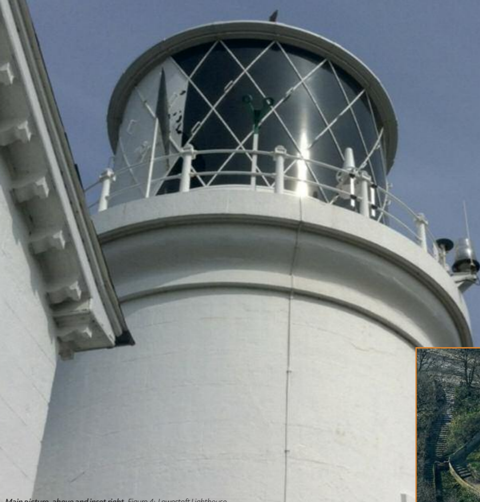
Main picture, above and inset right, Figure 4: Lowestoft Lighthouse.
