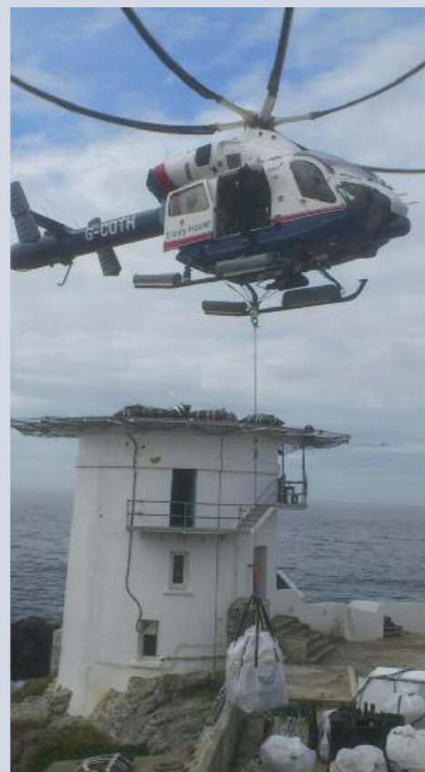
Above: Helicopter underslinging operations.
