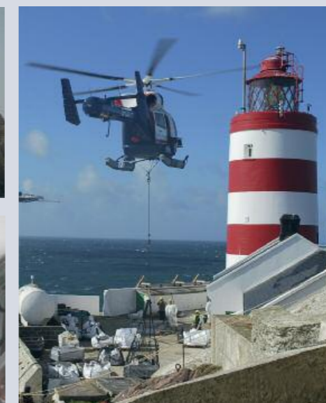
Above: Helicopter underslinging operations.
