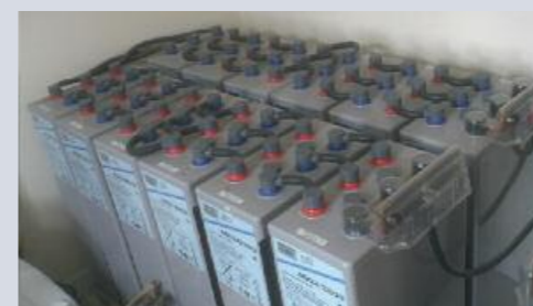
Above: Sealed gel batteries and racks.
