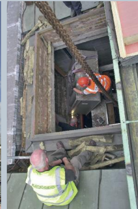
Above right: The unit is located in the roof top plant room which can only be accessed by removal of a section of the roof and via a small aperture in the structure.
