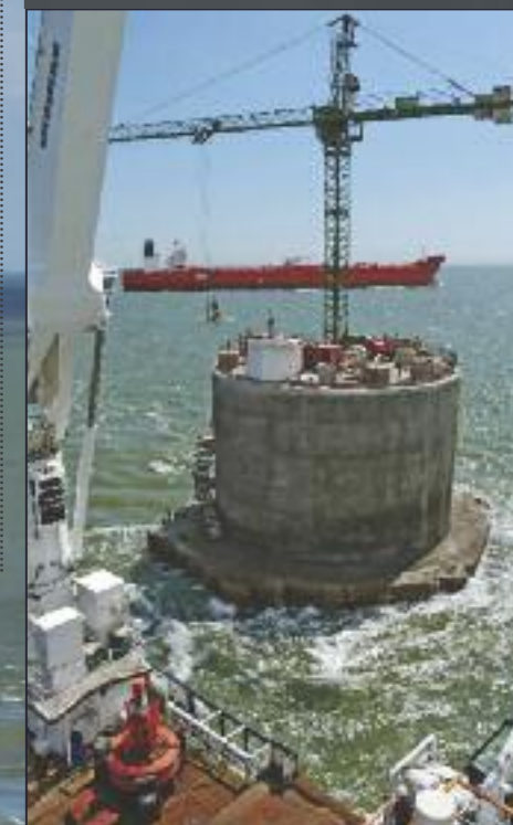
Above & below: July 2014 with THV Galatea craning on the refurbished pepper pot aids to navigation unit. Photograph ©Ambrose Greenway.
