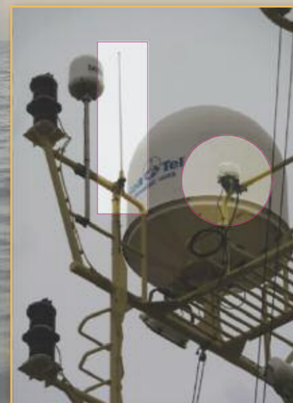
Figure 2: Close-up of the AIS AtoN installation on THV Alert.
