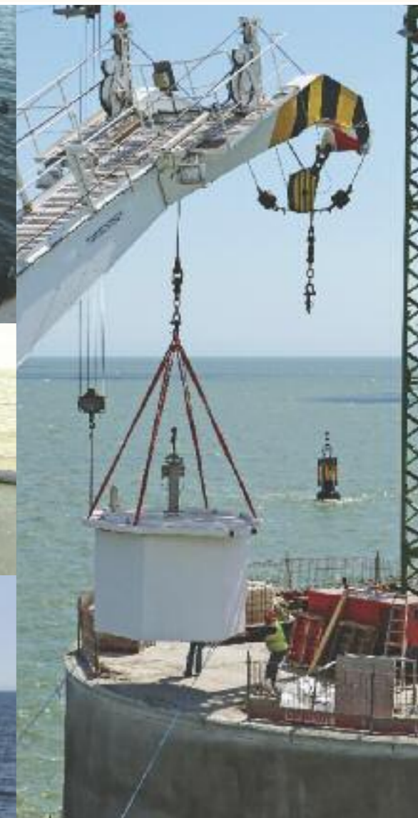
Top left: Securing a line on a buoy's tailtube. A high standard of safety is achieved by each vessel in the Trinity House fleet regularly reviewing safe systems of work in the form of standard operating procedures. © Trinity House Top right: Craning in the aids to navigation module during the recent Nab Tower refurbishment. Very close attention is given to the capacity of lifting gear and the means by which loads are secured. Photograph: © Ambrose Greenway Middle left: Releasing the shackle on a buoy sinker. Staff in the tenders work in the harshest of weathers and all year round ensuring safety of navigation for the world's mariners in our waters. © Trinity House Middle, lower left: The seemingly innocent unmanned and automatic lightvessel holds many surprises for the inexperienced with slips and falls on the bird-fouled decks, ladders to be encountered and safe entry to be effected to enclosed spaces. Photograph: Captain Roger Barker © Lower left: Where incidents or near misses occur, these are investigated, standard operating procedures reviewed and adjusted accordingly. © Frances Baskerville, CIRM
