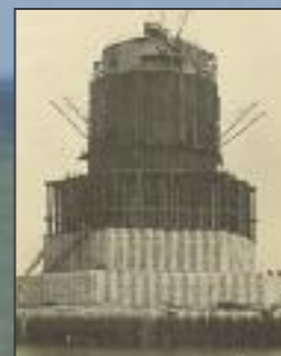
Nab Tower, built for the Admiralty in Shoreham from hollow concrete sections and steel in 1918.
