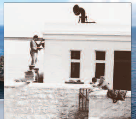
Under the direction of Sir John Bowen, Engineer-in-Chief from 1924 to 1951, the station was repaired following wartime damage.
