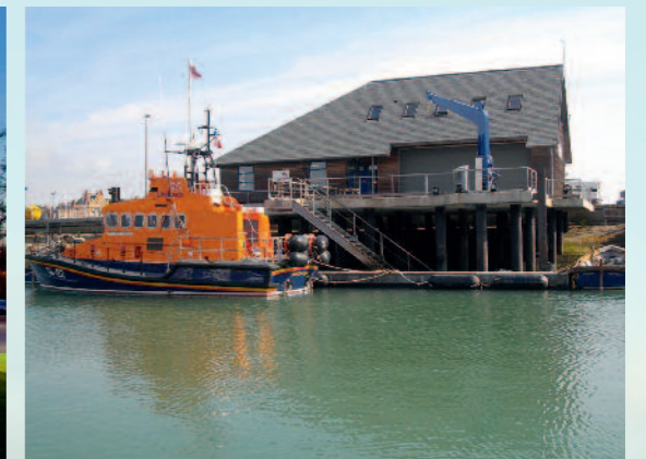
Above: The refurbished RNLI Station at Ramsgate.
