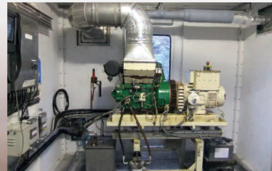
Above: The Lister TS3 engine as installed at Skerries lighthouse. A similar power unit operates at Hurst lighthouse.
