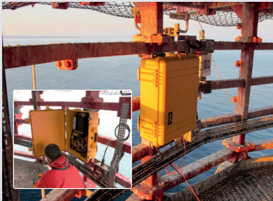
Above and inset: Ruggedised case containing video monitoring hardware fixed to the helipad support structure. Photos: © Tony Tapp.
