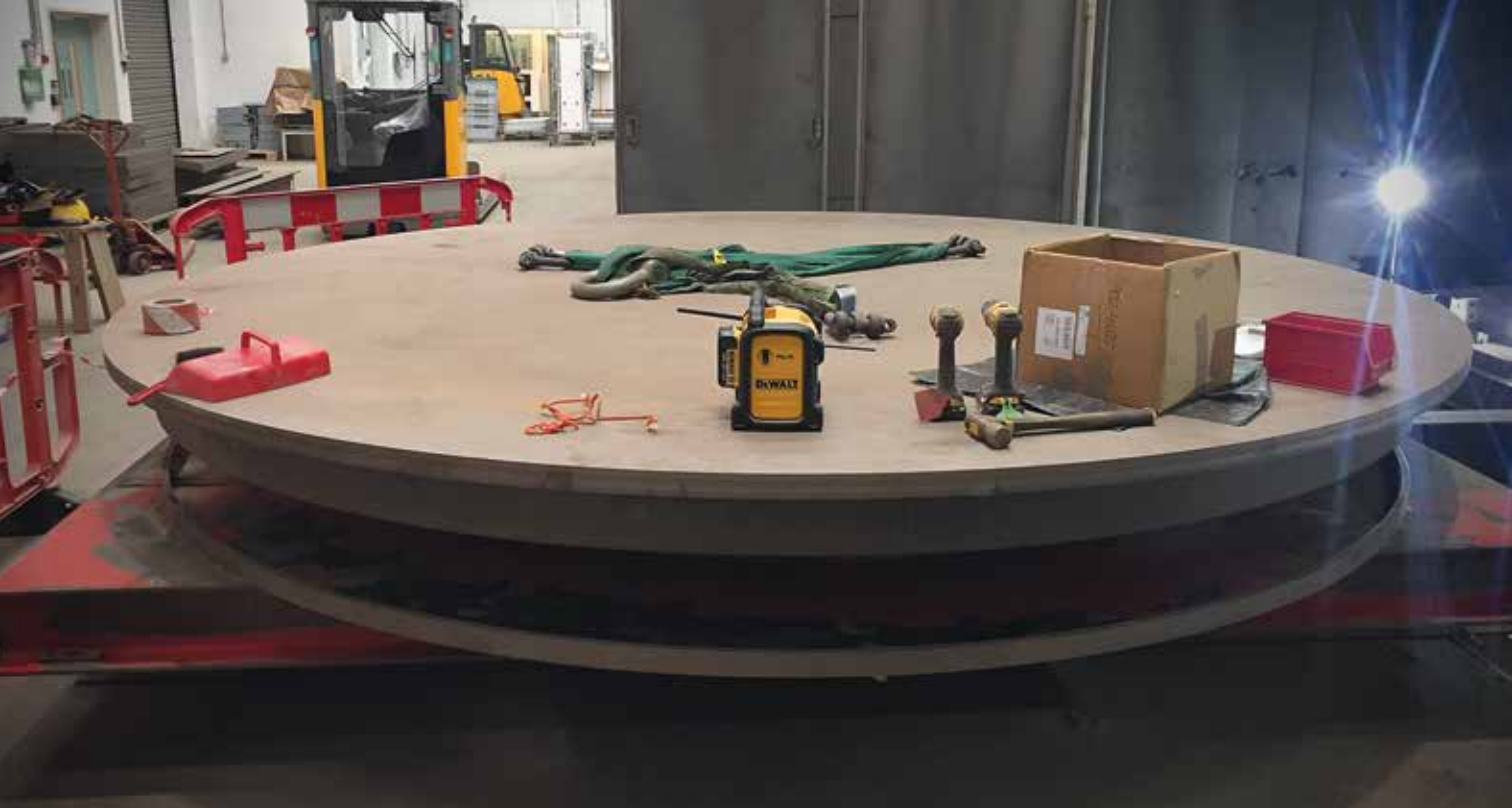
Installing the new turntable
