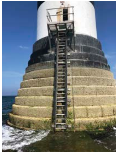
New access ladder and platform
