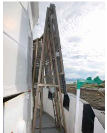
Installation of new larger solar frames
