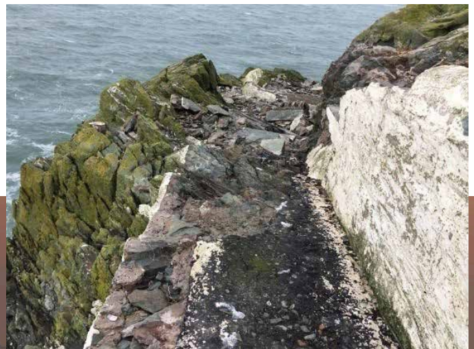
Top: Pre-storm; above: Post-storm
