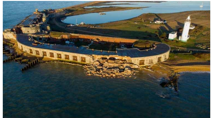
Figure 7: Impact of storm events of Hurst Castle.
