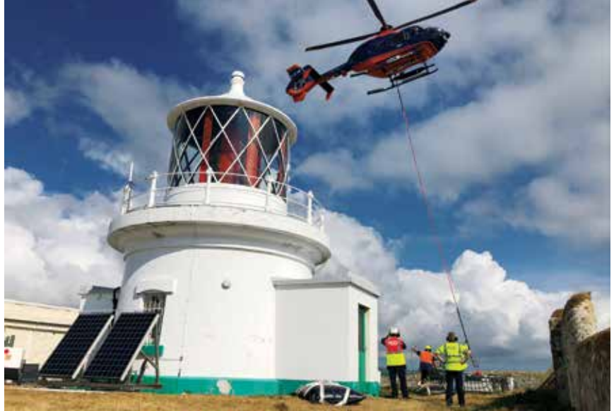
Landing supplies at the lighthouse
