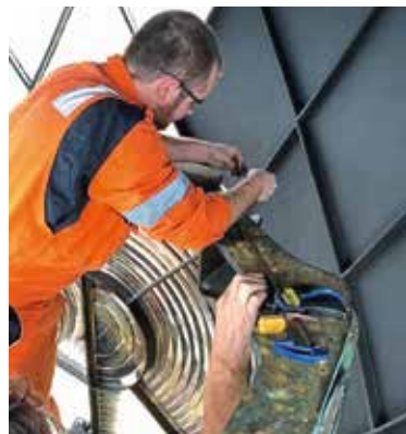
◀ The team disassembles the historical optic (seen above) to make way for the new LED lantern.
