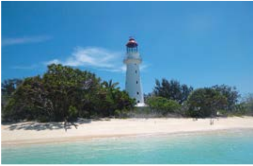
◀ North Reef Lighthouse (Queensland) built 1878 (AMSA 2020)
