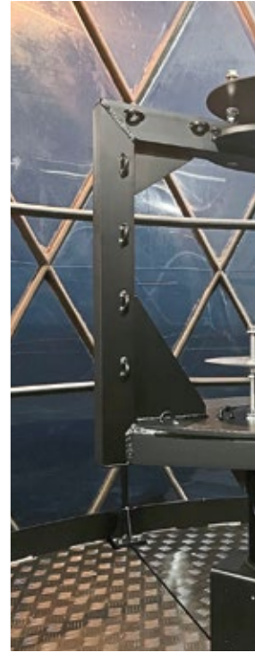
► Pendeen Lighthouse's new light pedestal
