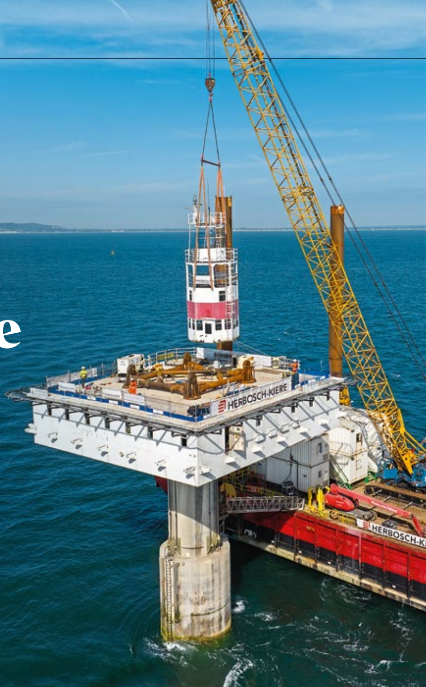
▲ Royal Sovereign Lighthouse lantern tower being lifted by Gulliver
