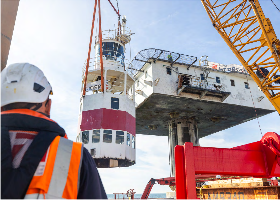
Removal of Royal Sovereign Lighthouse's topsides in October 2023
