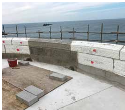
▼ Parapet blocks refitted following repairs to tanks
