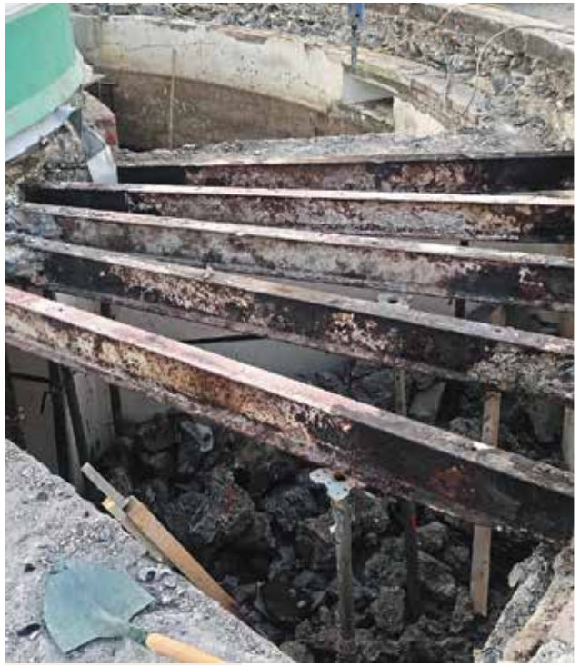
▲ Beams of the tanks undergoing repairs
