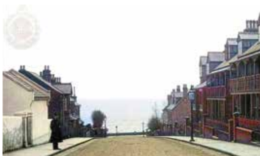
▲ Beach Road showing the extant Donkey House (Store) on the left of the photograph © Harwichand Dovercourt.com
